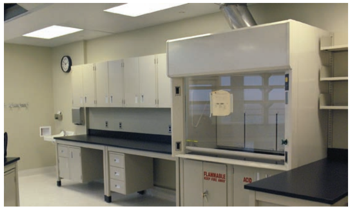
A neuropharmacology lab at Health Sciences Centre, built from scratch by Westland Construction in 2008.
