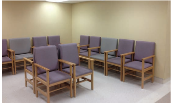
A waiting room in Concordia Hospital's diagnostic imaging area. Westland Construction built the room and modified nearby office space in 2013.
