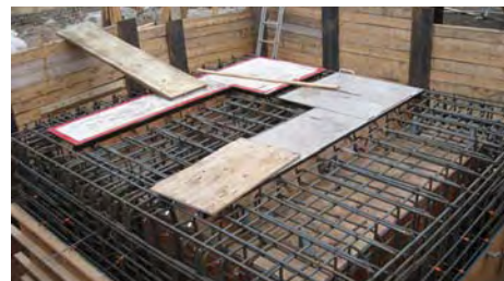
The overflow chamber in progress: the walls are seven metres high and 16 inches thick.
