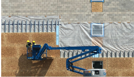
Installing insulation and firewall
